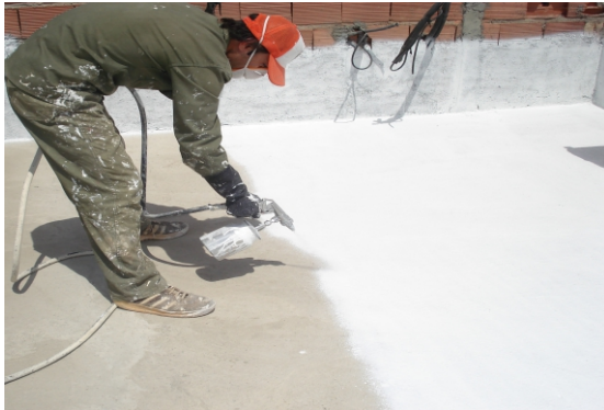
Pictures during painting work
