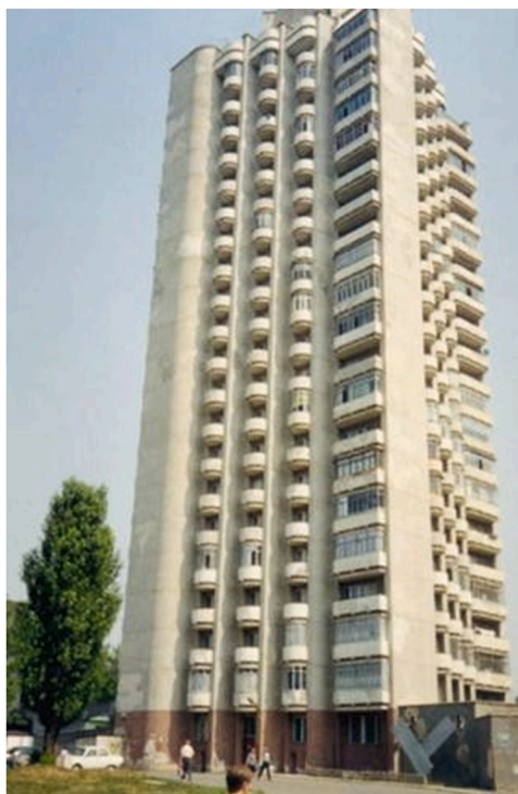
Fig. 12. The first residential building made of alkali-activated concrete without any OPC was built in 1989 in Liepstk, Russian Federation [174].
